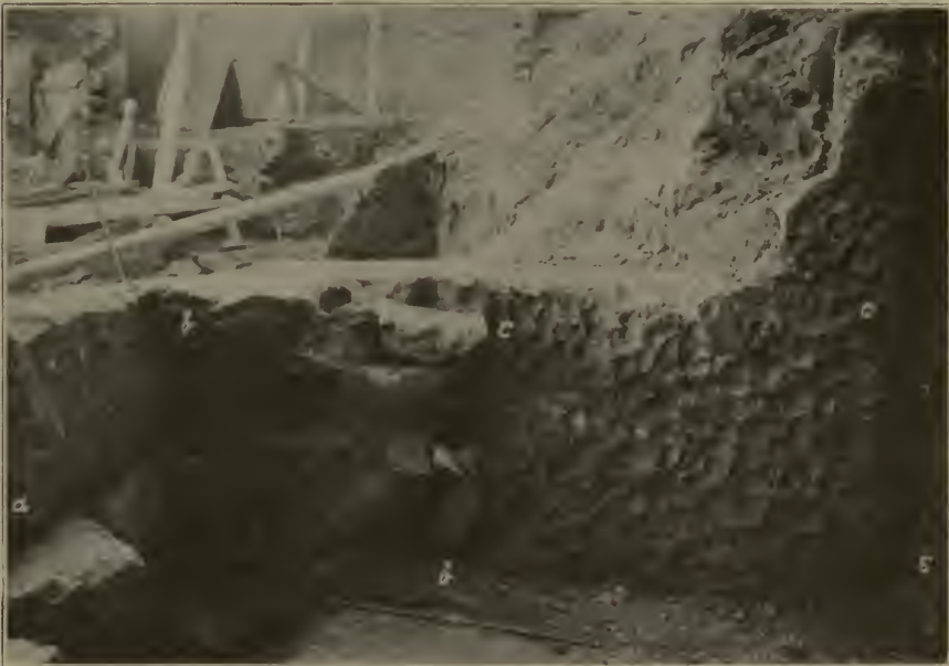
FIG. 6.—ROMAN WALL (INTERIOR, LOOKING SOUTH). a Inner face of ashlar work ; b Rubble ; c Clay-loam backing ; d Made earth.
